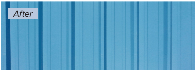
Manufacturing Facility Treated With X-RESTORE Oxidized Metal
